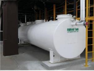
Passive Grease Interceptors With Exclusive Switchback Baffle System
