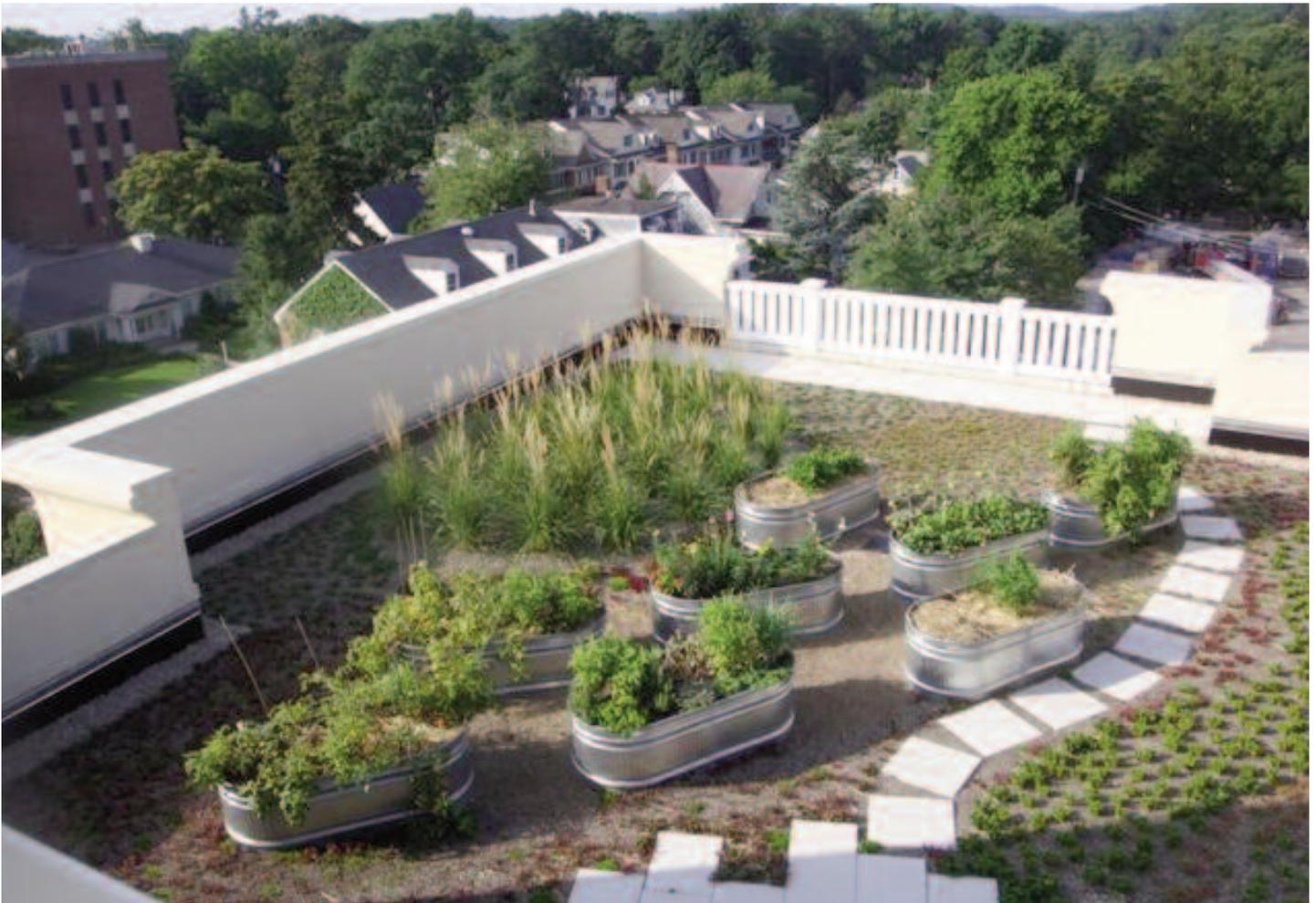
A vegetative roof reduces solar heat gain and improves water quality flowing from the roof of a green office/parking garage in Morristown.
