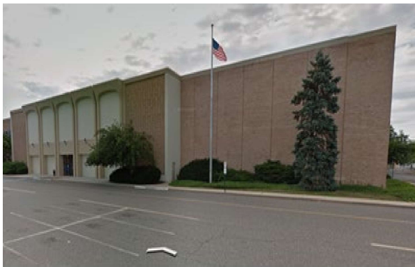
The former Sears building located at the Moorestown Mall, Moorestown, New Jersey.
