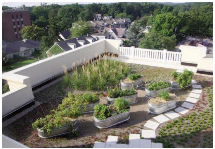
A vegetative roof reduces solar heat gain and improves water quality flowing from the roof of a green office/parking garage in Morristown.
